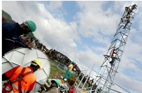
*Technicians assemble the pieces of the cell tower. Due to the difficulty of accessing rural towns, implementation of the solar stations needs to be completed in a single visit.*
